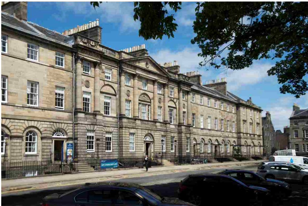
Figure 24. The north side of Charlotte Square in 2013 with leftmost dormer removed. Source: D. Henrie.
