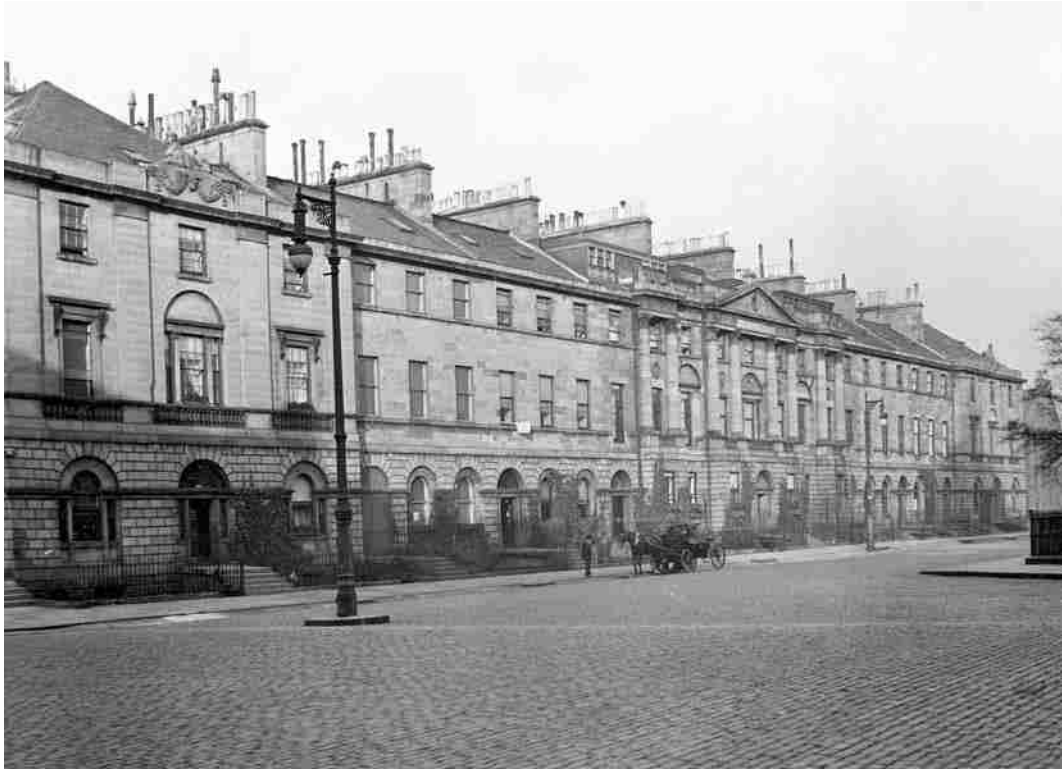
Figure 23. The north side of Charlotte Square in c.1890. The dormer at No. 7 is visible to the left and above the leftmost column. Source: RCAHMS 130 1728.
